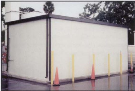
BOOTH INSTALLED IN PARKING LOT TO SAVE SHOP SPACE
